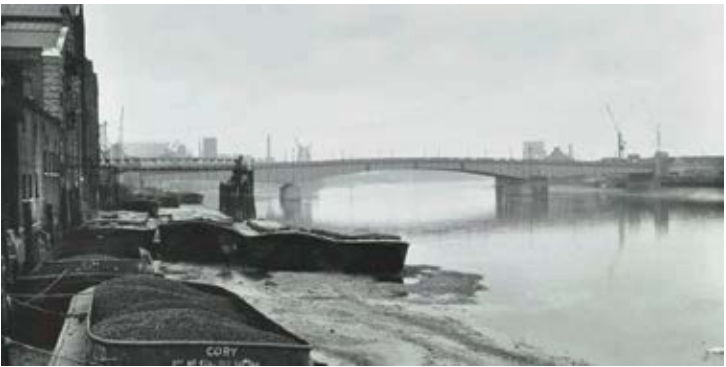
Battersea Bridge, a five-span arch bridge over the River Thames in London, opened in 1890.
